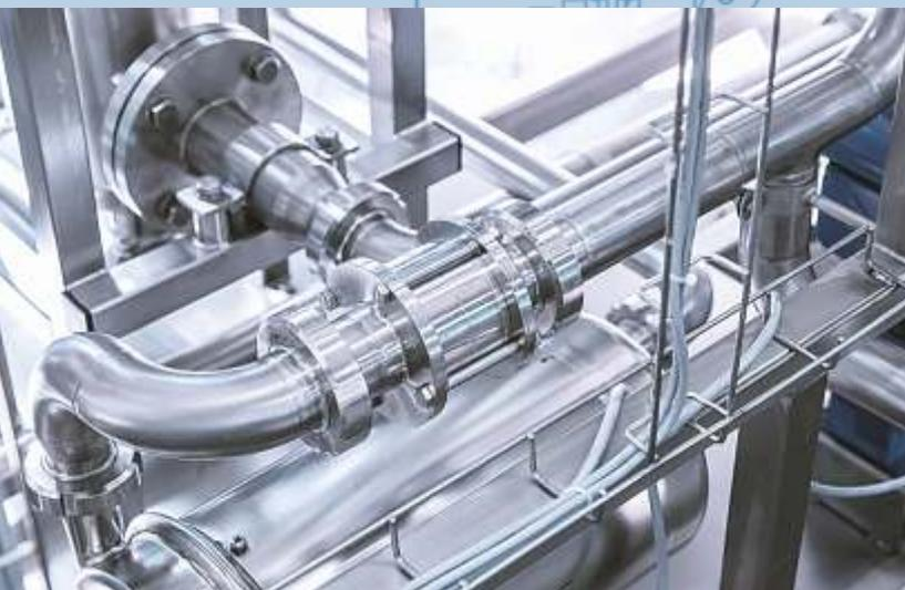
**ENG** The pumping station consists of a main pump and three auxiliary pumps that control proportions of alkaline, acidic and disinfecting agents. Valves are provided to control the flow of water and cleaning agents.
